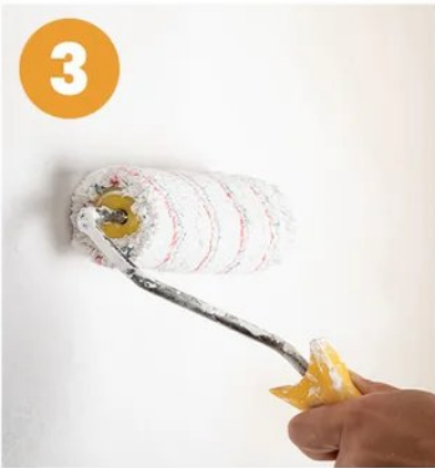
APPLY EVENLY Maintain a wet edge and apply a uniform coat. Avoid overworking the paint.
