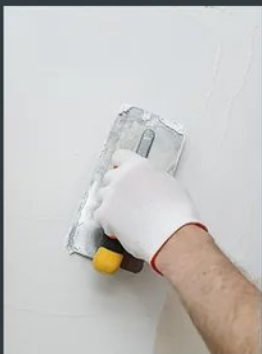
PLASTER & PATCHED SURFACES
