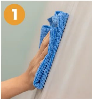
CLEAN & PREP Remove dust, grease, loose paint and any contaminants. Repair imperfections and allow surfaces to dry.
